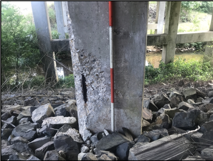
Bent 2 column 2, large spall with exposed rebar with section loss.
