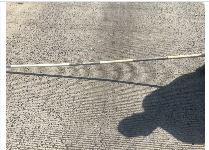
Deck span 5 has longitudinal unsealed crack that reflects through to the soffit.
