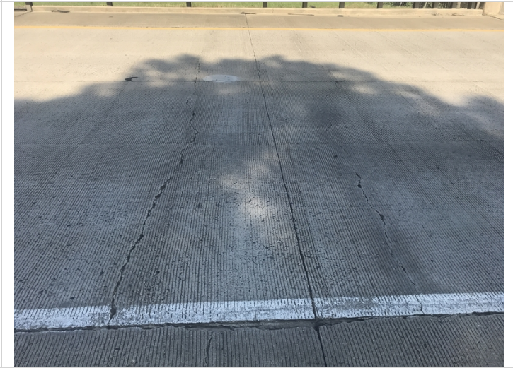
West approach slab has large unsealed cracks.
