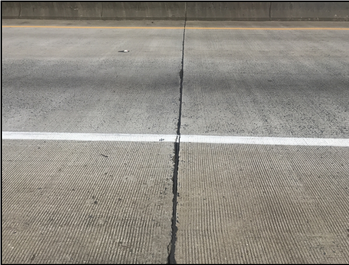
Bent 3, loss of bond and leaking.
