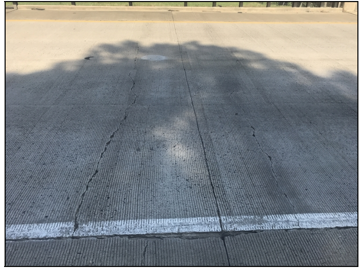
West approach slab has large unsealed cracks.
