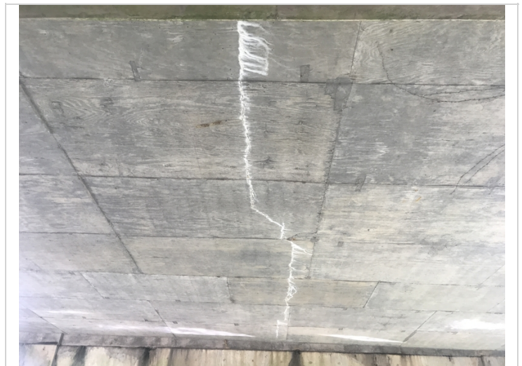
Span 2 soffit has cracks with efflorescence at centerline, common all spans.
