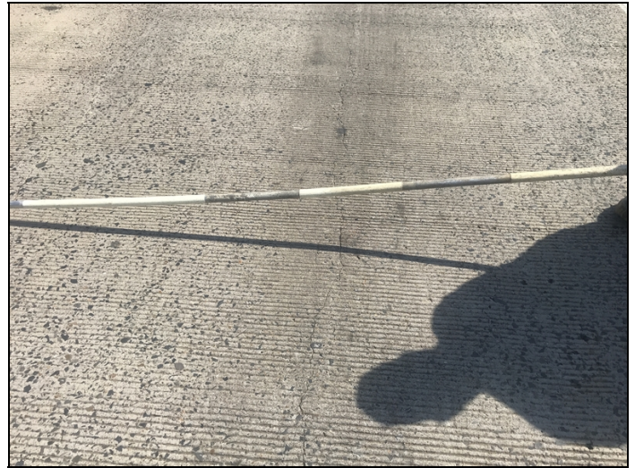
Deck span 5 has longitudinal unsealed crack that reflects through to the soffit.
