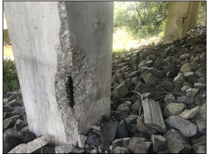
Bent 2 columns 2&3 have large spalls with exposed rebar.
