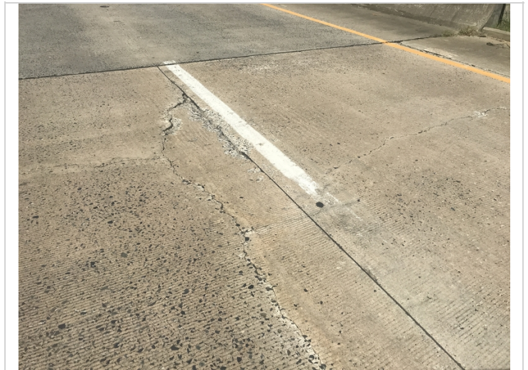
East approach slab has deep spalls.
