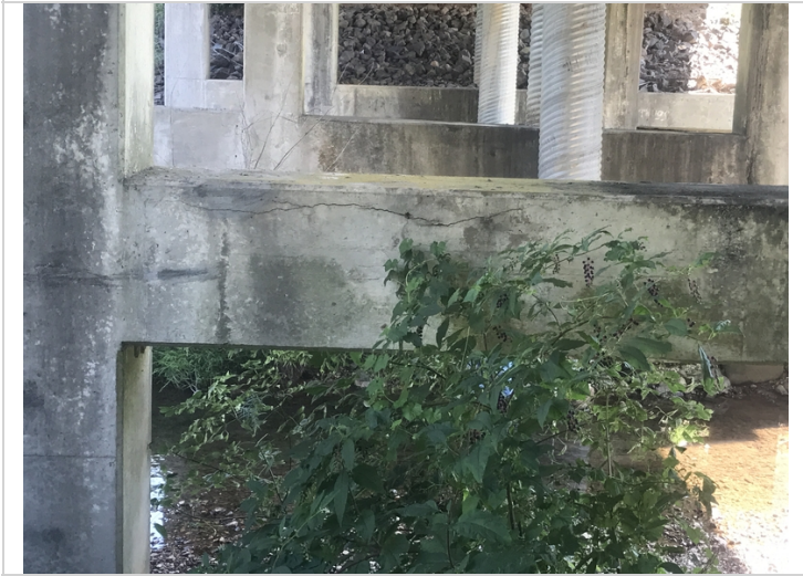
Pier wall (interior strut) at bent 3 between columns 2&3 has crack.
