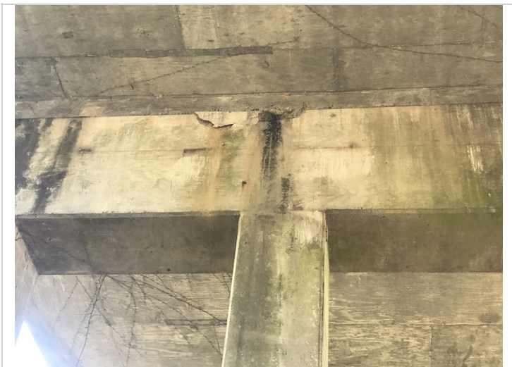
Bent 4 cap back has large delam.
