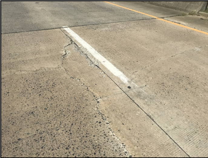
East approach slab has deep spalls.
