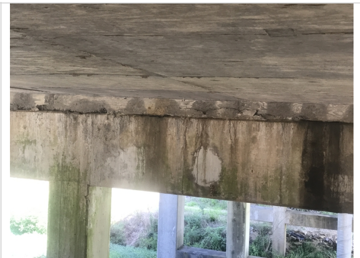
Deck haunch at bent 2 has spalls and delams.
