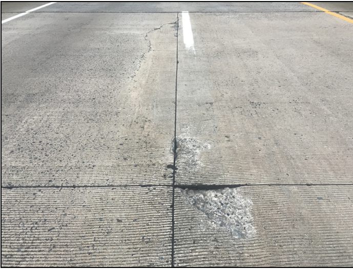
Large spalls and large cracks in east approach slab.
