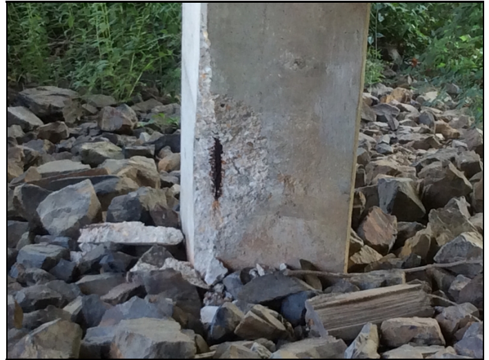
Bent 2 columns 2 and 3 have large spalls with rebar exposed
