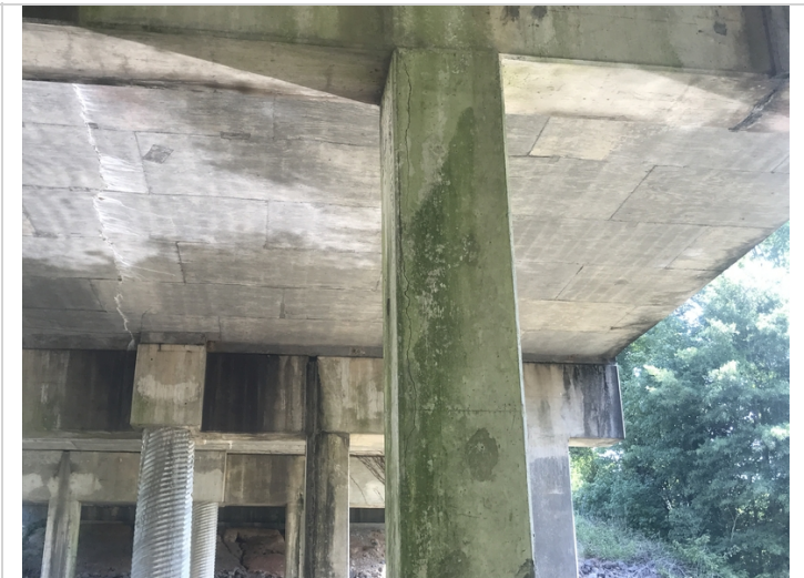
Bent 3 column 3 has crack.
