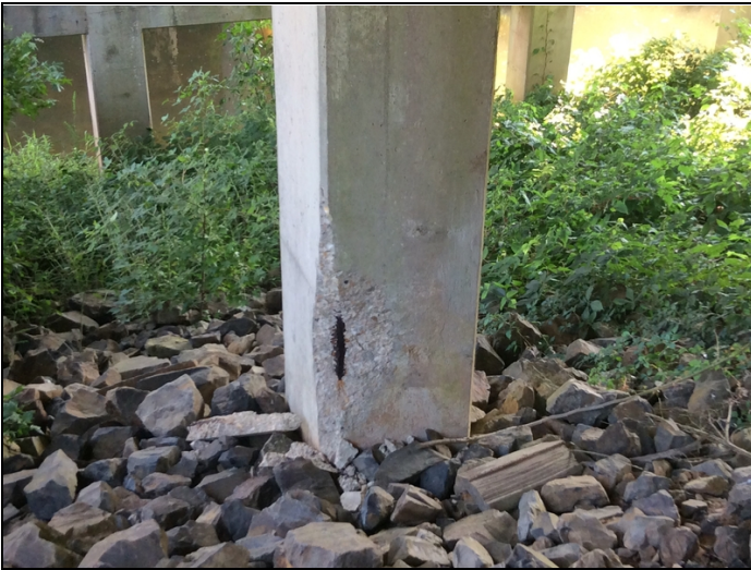
Bent 2 column 2 spall with exposed rebar
