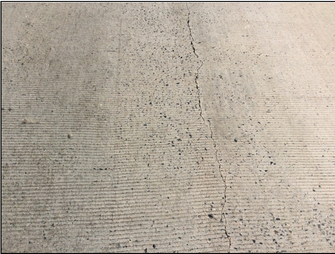
Deck has large unsealed cracks.
