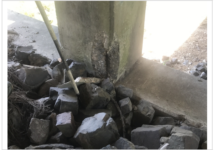
Bent 5 column 5 has large spall with exposed rebar.
