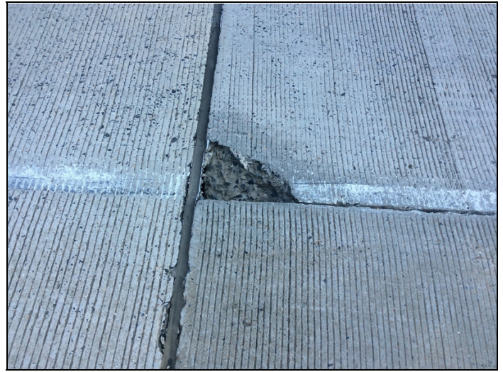
Approach slab at abutment 1 has a deep spall and unsealed cracks.
