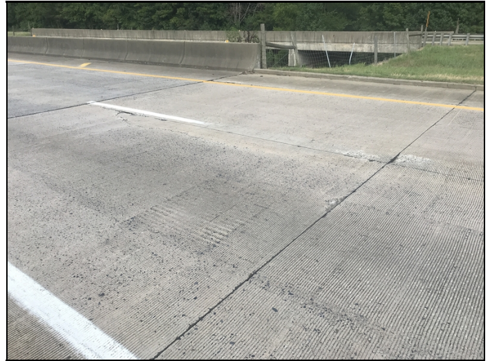
Large spalls and large cracks in east approach slab.
