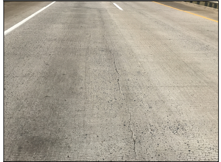
Span 1, large unsealed longitudinal crack.
