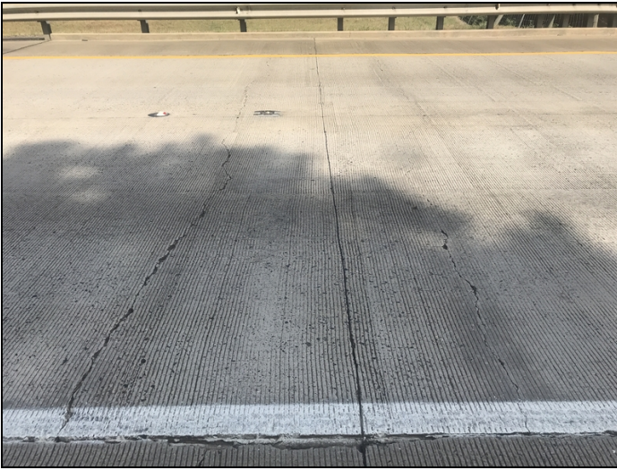
West approach slab, large cracks.
