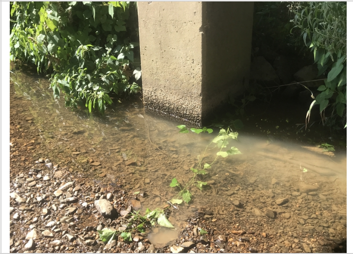
Bent 3 column 3 has abrasion at water line, common column 2.
