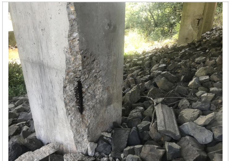
Bent 2 columns 2&3 have large spalls with exposed rebar.
