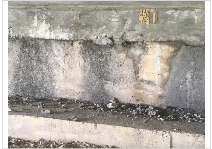
Bent 6 abutment patched area is spalling.
