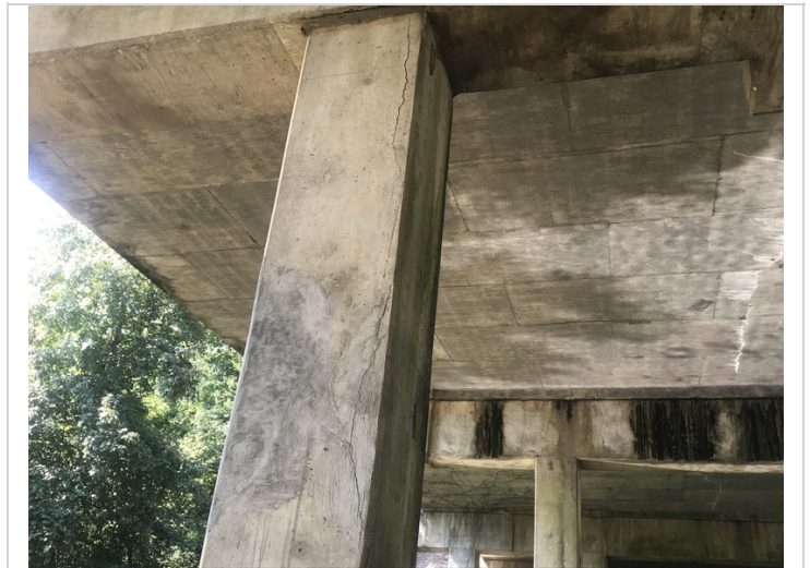
Bent 4 column 5 has crack.
