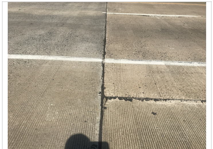
Bent 6 joint seal has lost bond and is leaking, common all joint seals.
